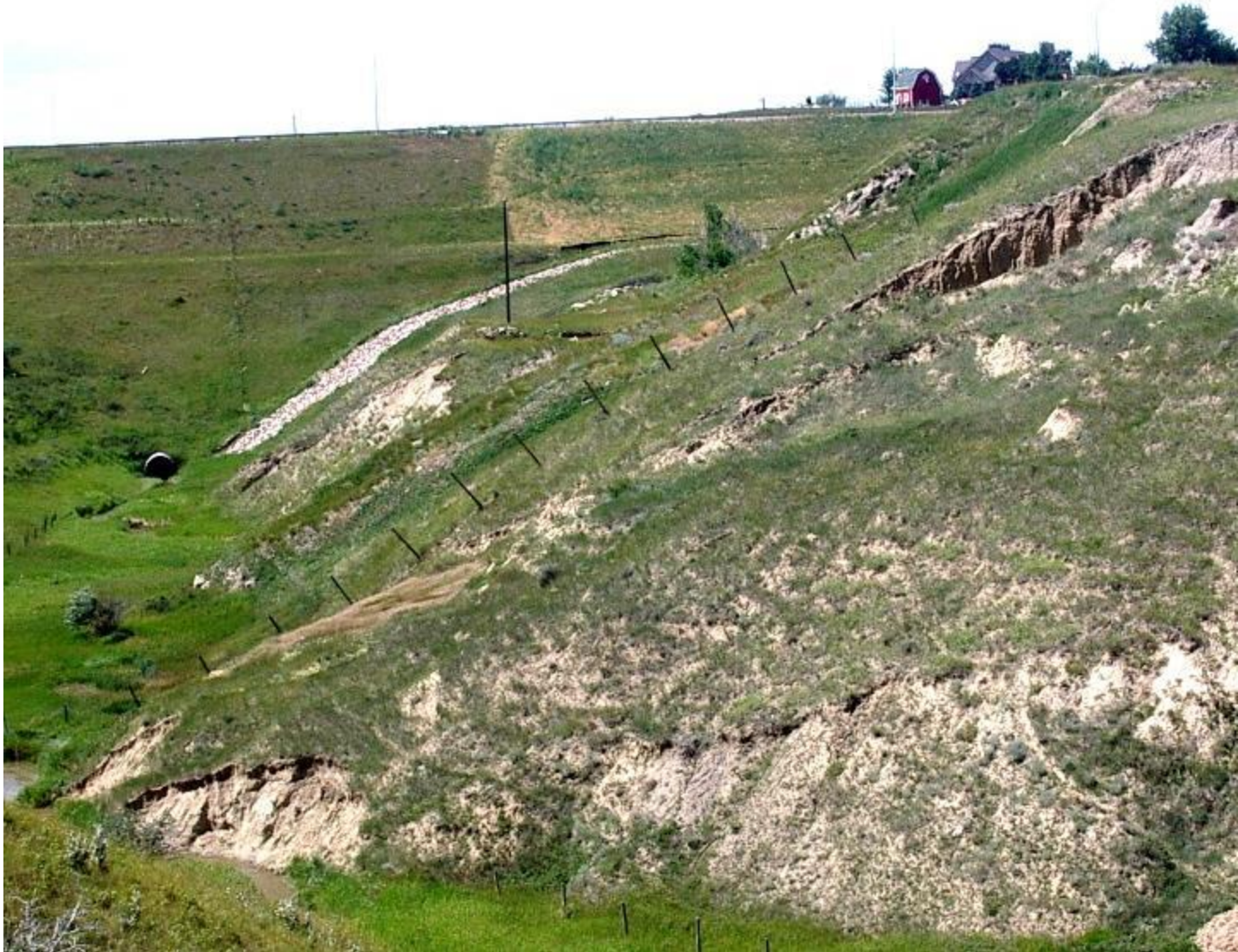
A slump. The main head-scarp is clearly visible at the top, and a second smaller one is visible about one-quarter of the way down. The toe of the slump is being eroded by a seasonal stream. S. Earle, CC-BY
