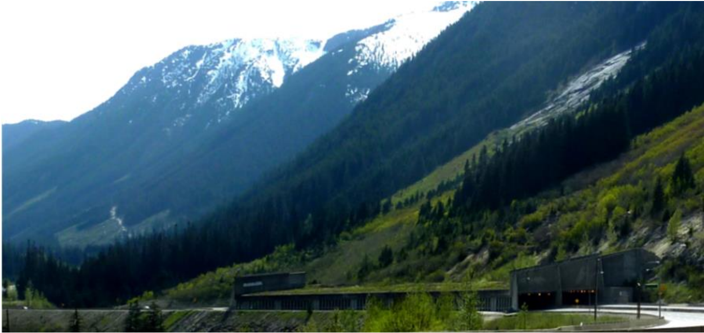
Figure 7.3.4 A snow avalanche shelter on the Coquihalla Highway, B.C., Canada. The expected path of the avalanche is the steep un-treed slope above. S. Earle, CC-BY
