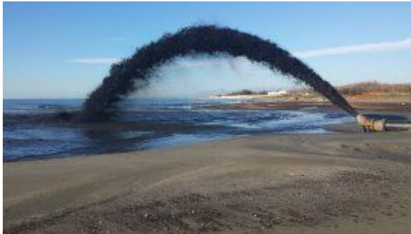
8.6.4 Sand dredging pumping sand back to the beach.
