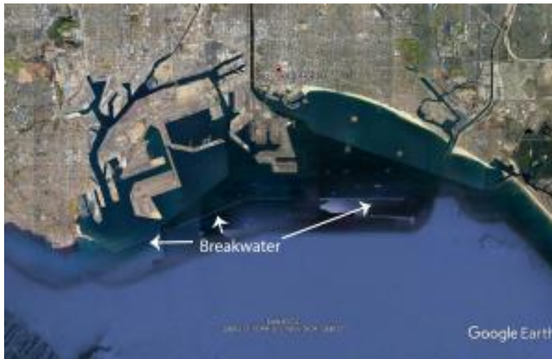
Figure 8.6.3 Breakwater off Long
